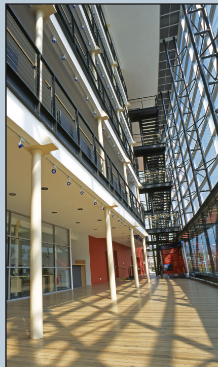
Kilncraigs Business Centre, Alloa. Above: cast-iron columns are retained internally behind the glazed curtain wall constructed in 2000. Below: A 19th-century woollen yarn store was skilfully extended in contrasting concrete and steel (left-hand side of photo) in 1938 by William Kerr. Most of the very deep original but multi-phase block (right-hand side of photo) was cut back and a new curtain wall added to the existing structure in 2000, making an assertive but revealing contrast of new and old, and achieving a visual link between Alloa Tower and the town. Junctions are clearly formed in red and white.
