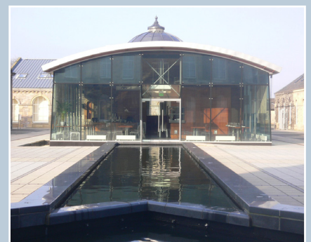
The extension to Esk Net Mills, Musselburgh, East Lothian. The glass extension of 2006 makes a deferential contrast to the solid masonry of the surrounding courtyard buildings of the 19th-century net-making complex. The design draws on the symmetry and scale of the old buildings, whilst creating a distinctive new component in its form and materials.
