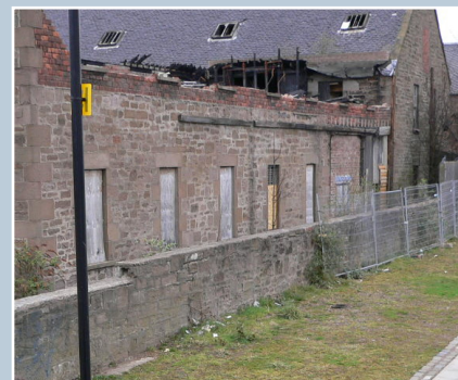
Former Arctic Tannery and Harbour Workshops, Dundee. A fire destroyed the upper part that had originally been of timber louvres to cure sealskin hides, replaced in brick. The development of housing (see below) echoes in a new form the timber and brick previously used here.
