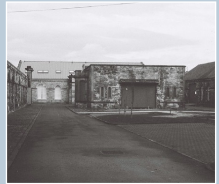
Esk Net Mills, Musselburgh in 1996 before refurbishment and extension.
