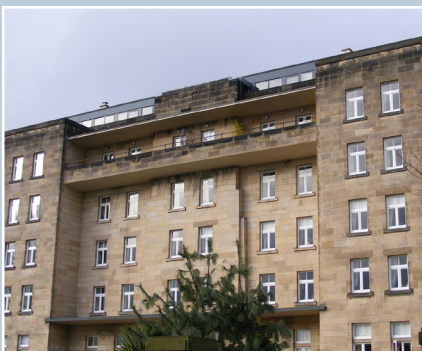
Former nurses' home of 1938–47, Salisbury Road, Edinburgh. The additional rooftop storey is set back from the wallheads, minimising its impact on the original design.
